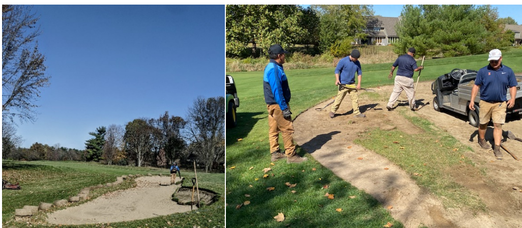
Bunker restoration in progress
