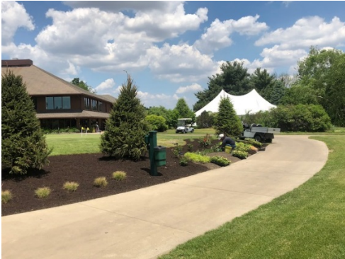
New landscape area at #10 tee/practice green in progress.
