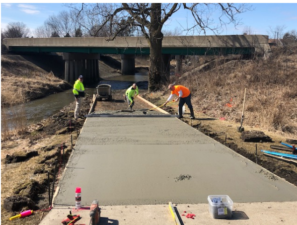
New path under I-57 in progress
