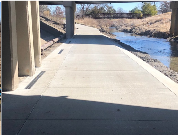
New path complete (Mayfield Construction)
