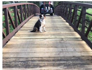
Earl checking our progress on bridge deck
