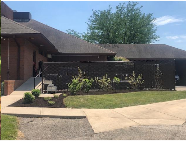
Loading dock landscape project
