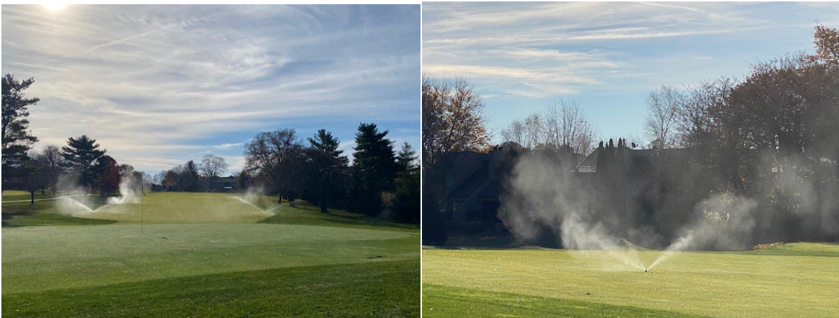
Irrigation blowout underway
